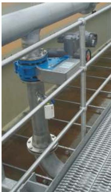
**IRIS diaphragm control valve with integrated air/gas flow measuring system ABB Sensyflow.**
